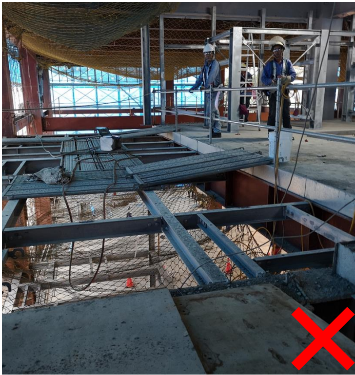
Unsafe: Platforms access to work areas do not have guardrail and lifeline
