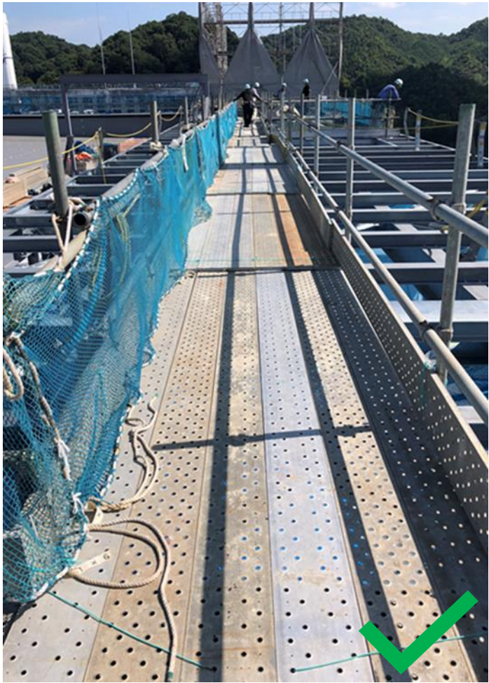
Best Practice: Proper walking platform with guardrails leading to the work areas
