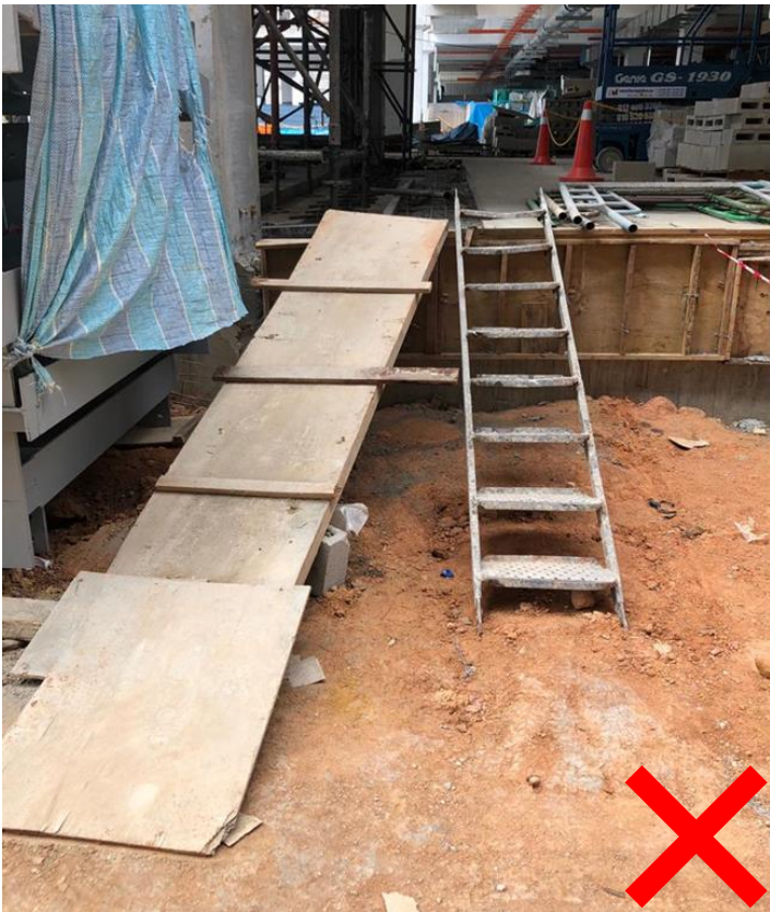
Unsafe: Makeshift timber platform and scaffold ladder used as access and egress
