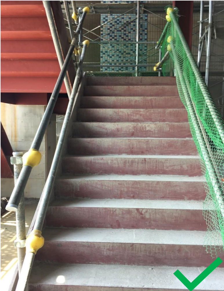
Best Practice: Stairway installed with proper guardrails and clear of tripping hazard
