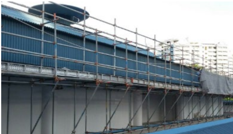
Figure 32 Cantilever Scaffold
